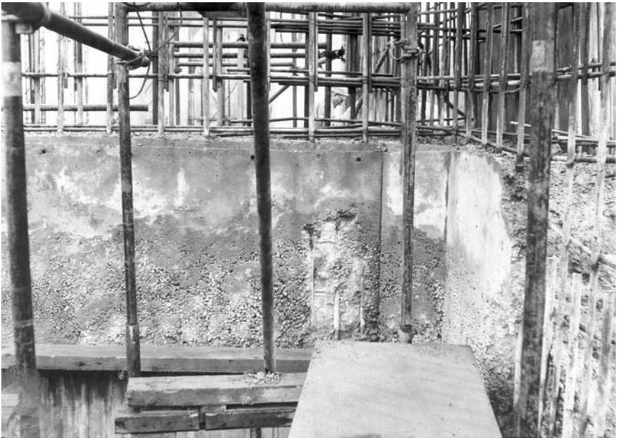
**Plate 16c.** Concrete which needs to be cut out: honeycombing and apparently inadequate cover to reinforcement
