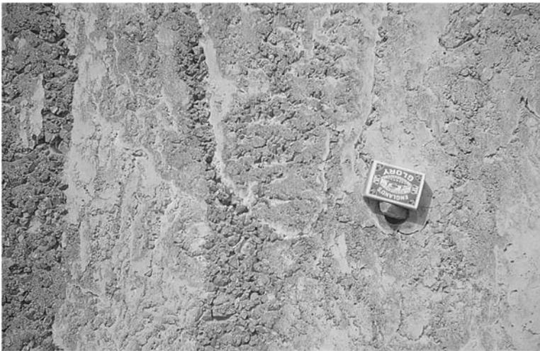
**Plate 15b.** Sand runs on a concrete wall surface
