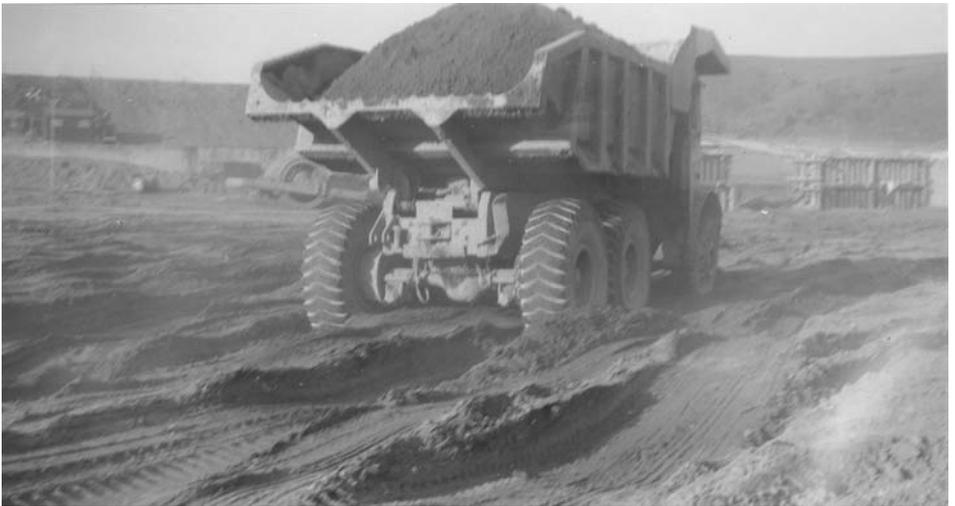
**Plate 4b.** A badly rutted formation, probably due to excessive moisture content of the fill
