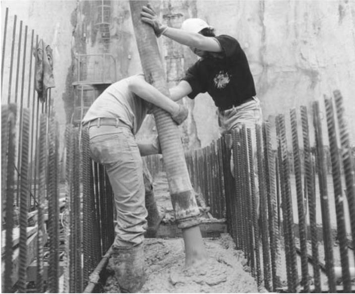
**Plate 14a.** The typical fluidity of pumped concrete; but it still needs vibrating in place
