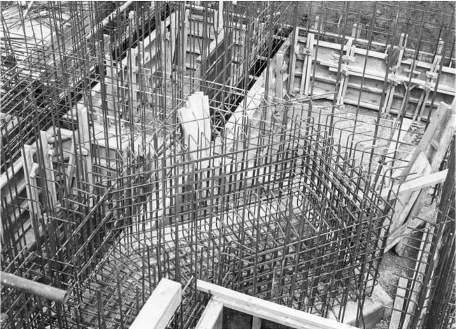
**Plate 14b.** Reinforcement must be accurately dimensioned and bent, and laps must be provided that permit the steelfixer to make adjustments for unavoidable discrepancies in the concrete work
